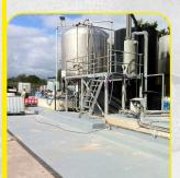
then protect all of the surfaces with a durable and highly acid resistant coating system. Therefore all of the concrete damaged by acid attack was broken out and removed, then thorough mechanical preparation of all of the concrete surfaces was carried out by blastcleaning.
